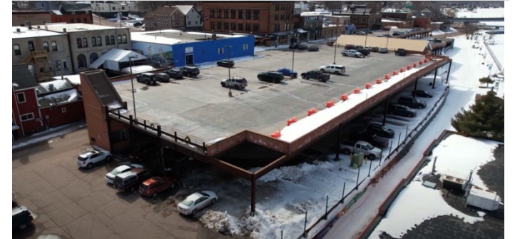
Demolish an aging parking deck
